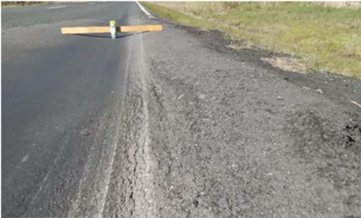
Figure 11: Pavement damage and deformation on Jingellic Rd (SWG business case)
